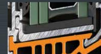
Special designed aluminium glazing support which transfers loads directly to the hinges, maximizing the functionality and the smooth operation of the sashes over time.
