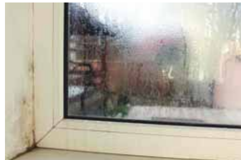
Figure 9.2B Formation of condensates and mold
