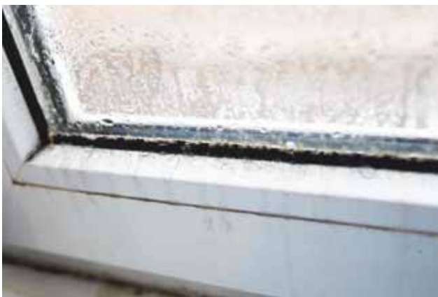
Figure 9.2B Formation of condensates and mold
