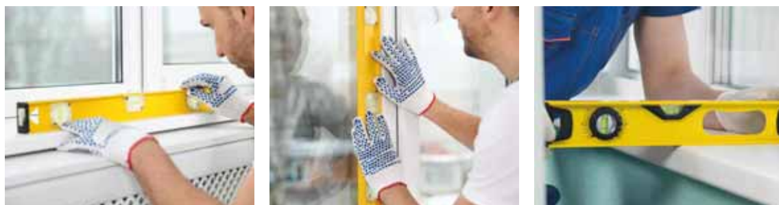
Figure 8.2.1 Vertical and horizontal leveling
