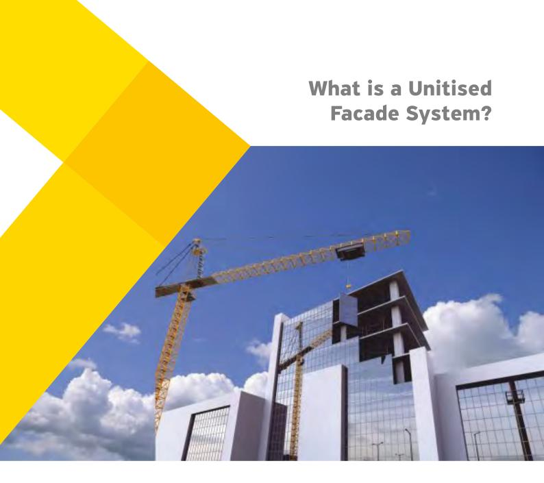
A unitised façade is a curtain wall system especially engineered for high-rise buildings. The construction of the building's envelope is done by assembling pre-fabricated units consisted of many frames, either structural or with visible aluminium covers.
